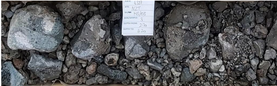
Slag-dominant Made Ground (d1), MADE GROUND: Grey, black and brown sandy angular and subangular fine to coarse GRAVEL of various lithologies including slag. With low to high cobble content. Cobbles and boulders are angular and subangular of various lithologies including slag, MS\BH08 core run 2.70m – 4.20m.
